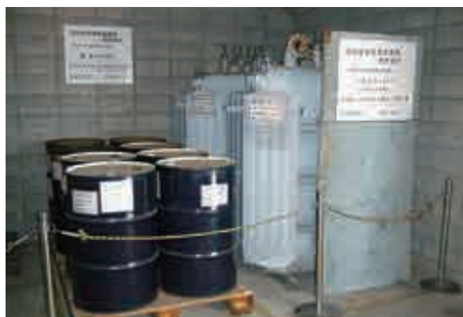
Low-contaminated PCB storage condition (Tokushima Production Div)
