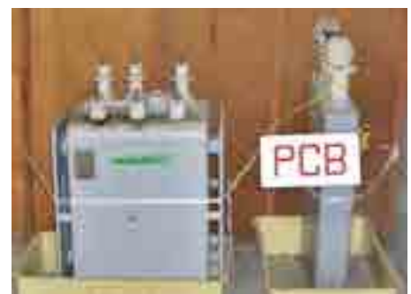
PCB storage conditions
