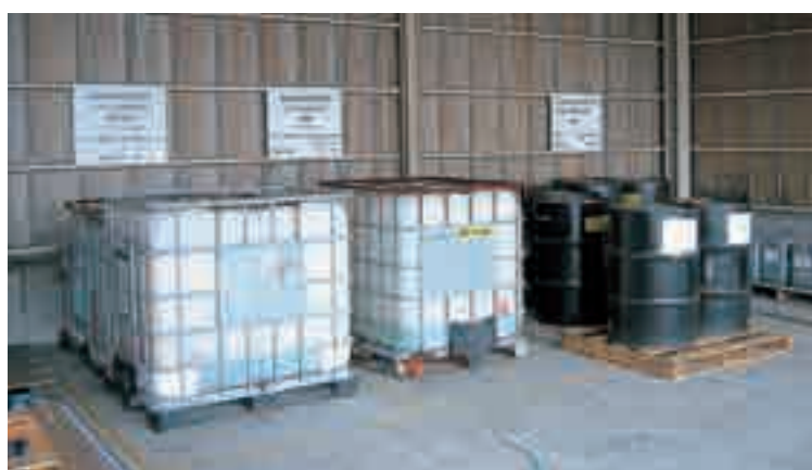
Tokushima Production Div. Designated waste liquid storage area
